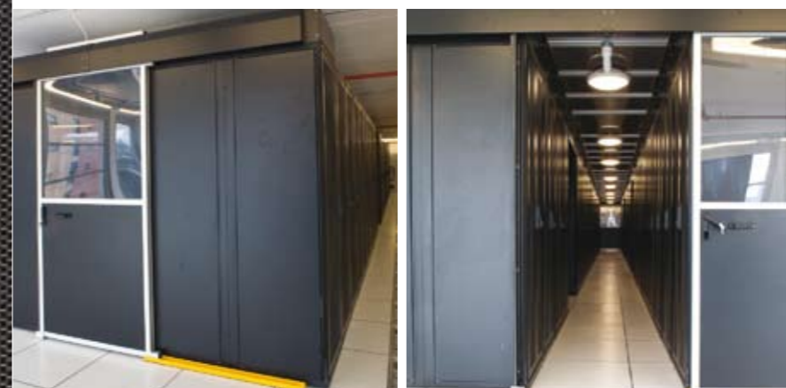
Fig. 6 CAE or HAE can be deployed in rooms with low ceilings.
